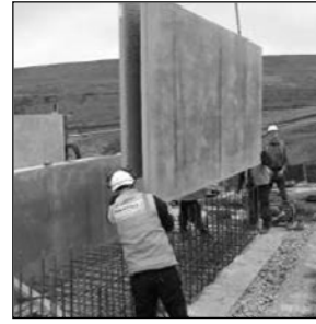
Figure 8. Oran Spillway Trial Panel
