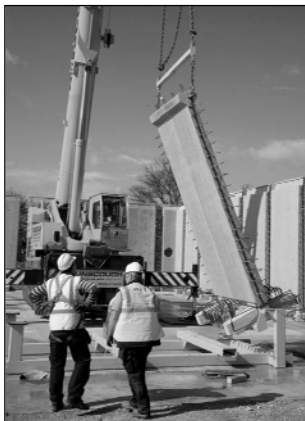
Figure 3. Installation of the precast units
