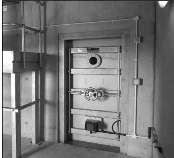
Figure 2. Pressure Door within pre-cast wall panel
