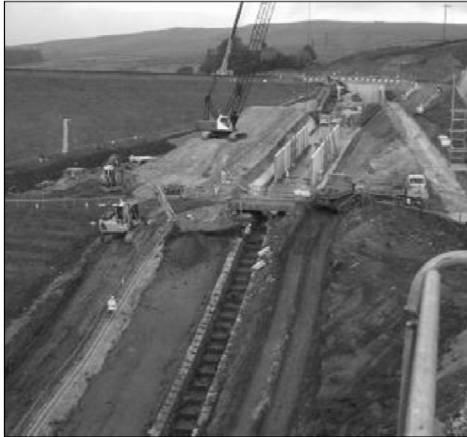
Figure 11. First reservoir precast spillway installation.
