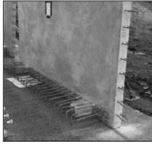
Figure 6. Carlow Spillway Trial Panel
