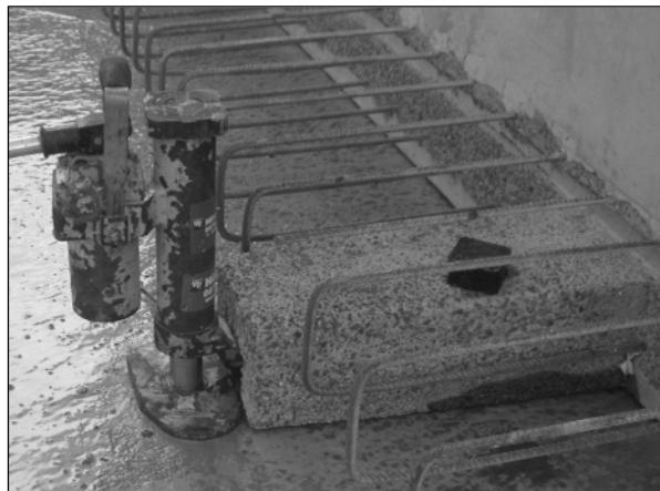
Figure 12. In situ wall joint to base level
