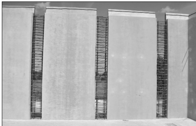
Figure 4. In situ wall joints under construction
