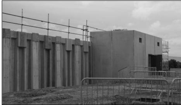
Figure 5. Completed Reservoir Structure
