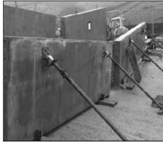
Figure 7. Whites Spillway Trial Panel
